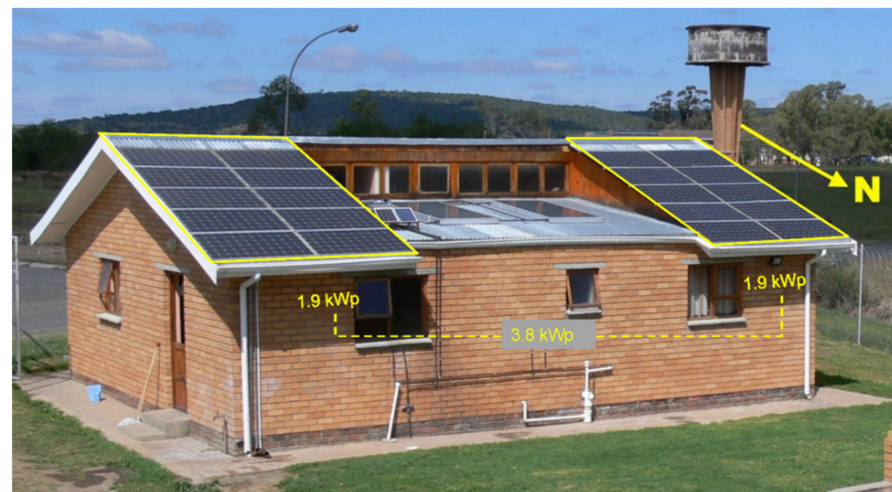
Figure 5. The case study solar photovoltaic system.
