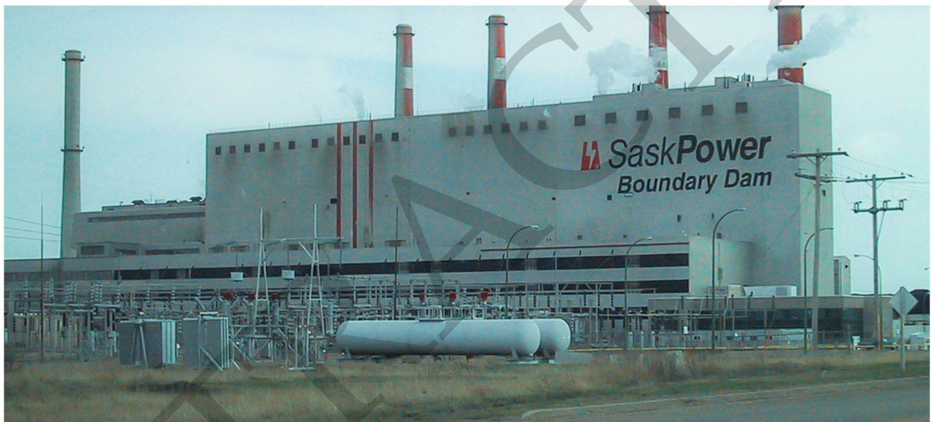
Figure 3. SaskPower carbon capture and storage project, Saskatchewan province, Canada. This project involves post-combustion capture of CO 2 accompanied with CO 2 -EOR [65].
