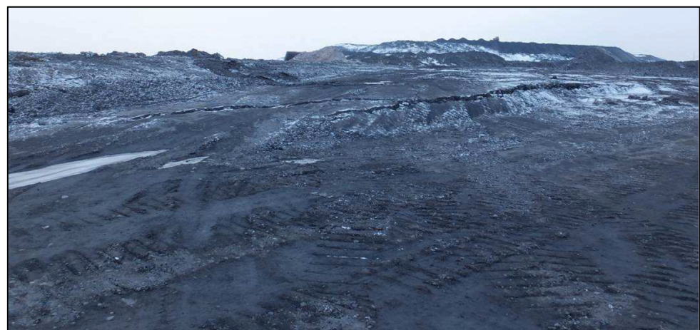
Figure 2. The failure observed on the surface of the Janina mine waste dump (10 February 2017).
