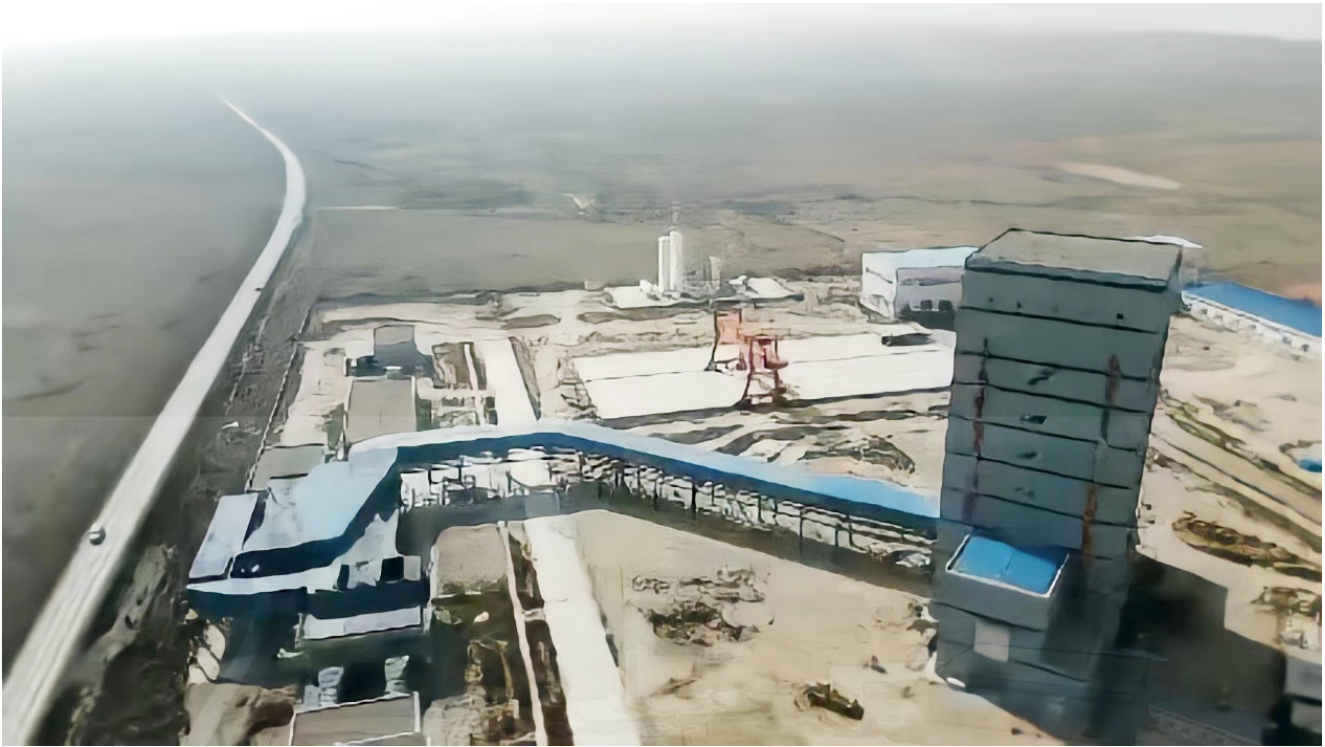
Figure 7. Engineering drawing of gravity heat pipe heat exchange project in a mine.
