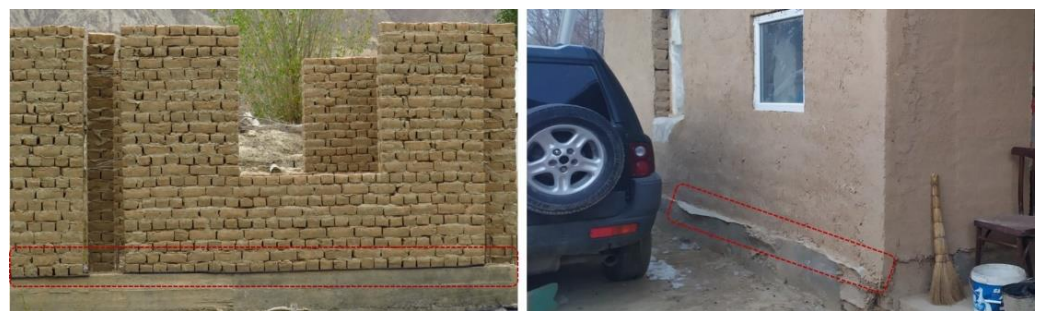
Figure 15. Provision of vapour barrier to avoid water diffusion on walls.
