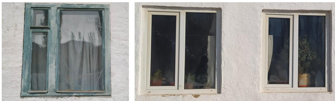
Figure 18. Traditional wooden windows (left) and newly installed PVC windows (right).
