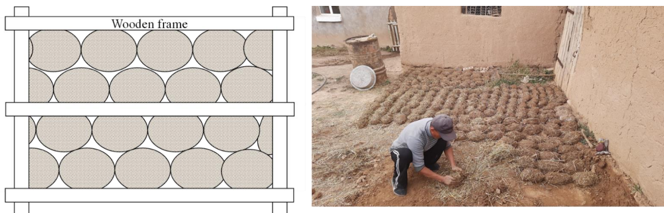
Figure 13. A wall structure with clay lumps and a wooden frame (left) and clay lumps in preparation (right).
