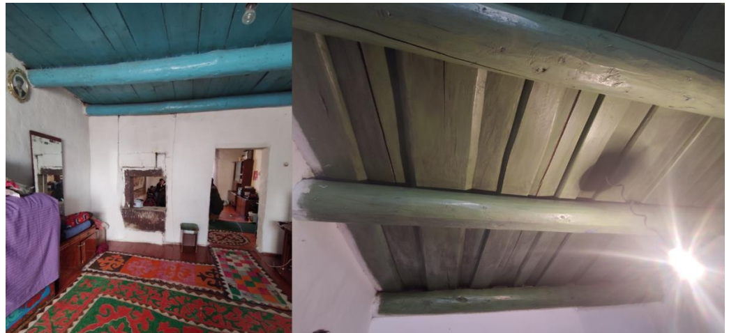
Figure 16. An example of a wooden-beam ceiling.
