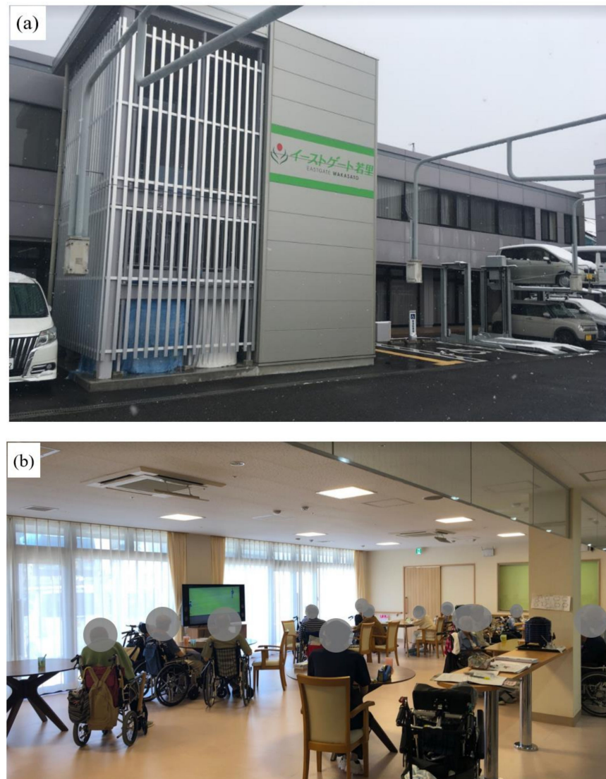
Figure 2. Survey objects: (a) survey building; (b) survey room.
