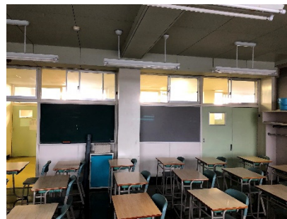
Ventilation window on the corridor side
