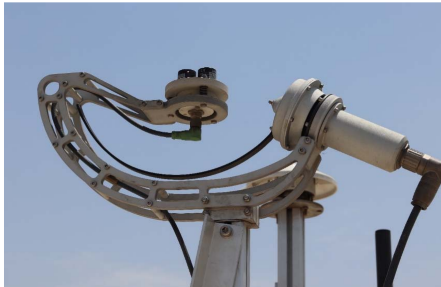
Figure 3. CSPC Twin-RSI installed at UET Peshawar.
