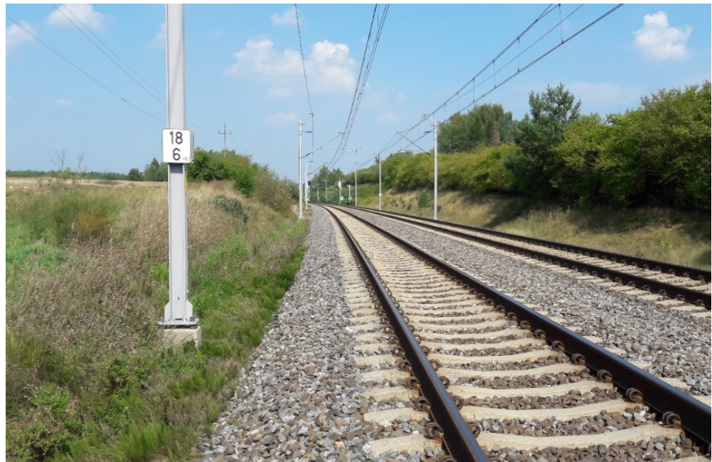
Figure 2. Railway track on the 18 + 600 km area of experimental research (a curve).
