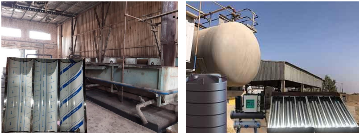
Figure 8. CPC collector system with high-temperature heat pump.
