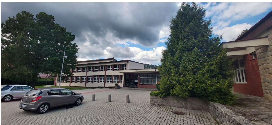
Figure 2. External view of the school before modernization.
