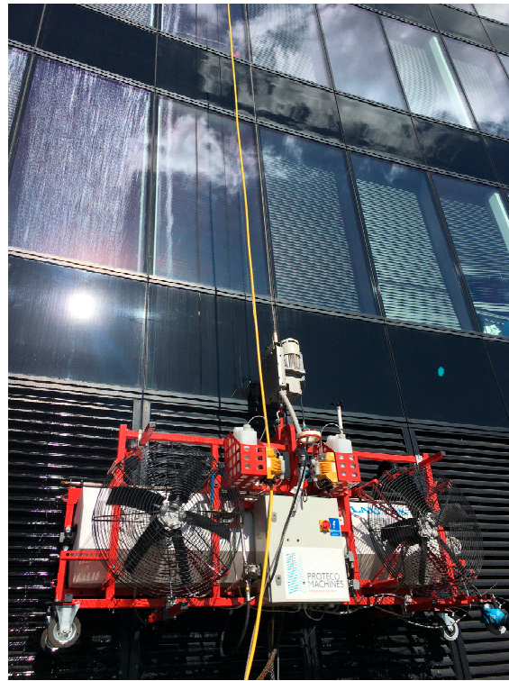
Figure 3. Facade washing machine before modernization [21].
