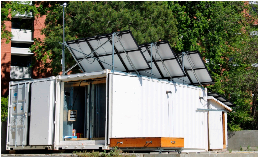
Figure 7. Overall photo of the completed test chamber from northwest corner.
