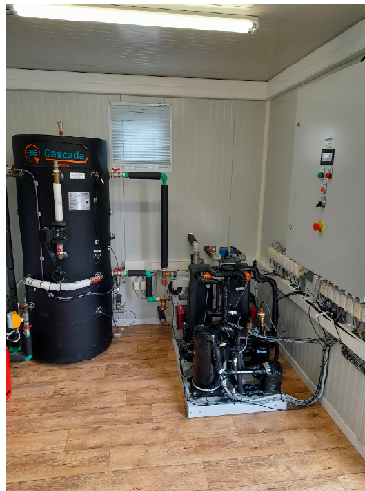
Figure 3. Heat pump and its electric/control panel in the control room next to the DHW tank.
