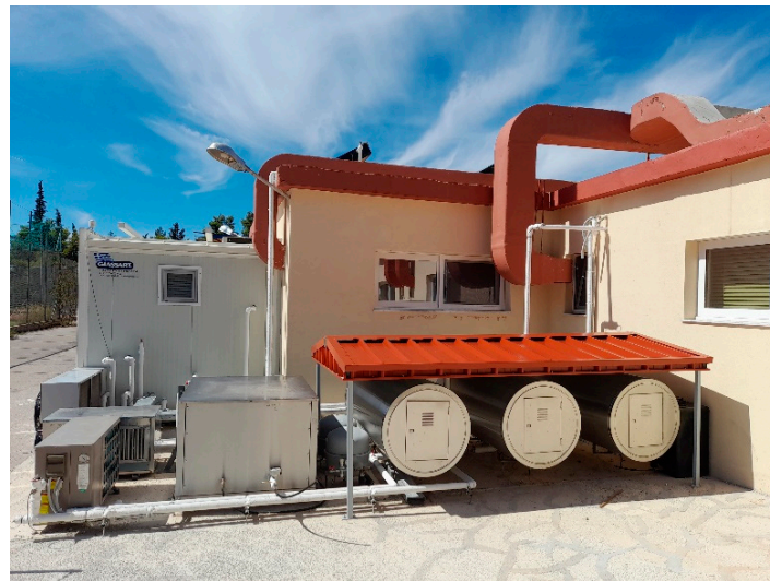
Figure 4. Outdoor horizontal water tanks under the shade. From left to right: virtual BTES, solar buffer, and space buffer tank.
