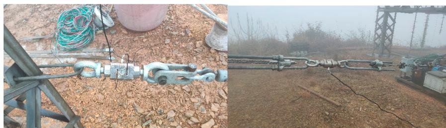
**Figure 3.** Suspension point of the test line.
