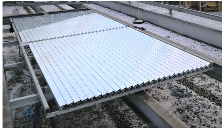
Figure 1. Fresnel mirror field at the University of Applied Sciences Upper Austria in Wels, Austria.
