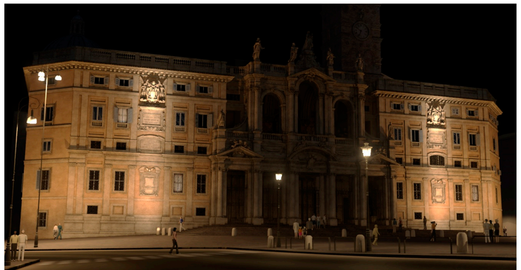
Figure 21. Visualization of the impact of street lighting with additional accent lighting on the basilica model facade.
