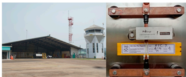
Figure 13. Installation of measurement system in tower near Air Traffic Controller.
