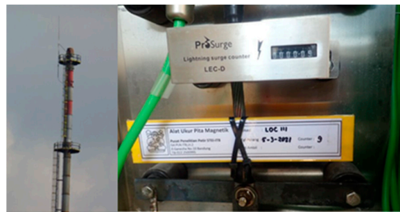
Figure 10. Installation of measurement system in stack structure.
