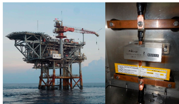
Figure 15. Installation of measurement system at an offshore facility.
