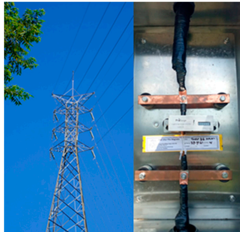
Figure 9. Installation of measurement system in transmission tower.
