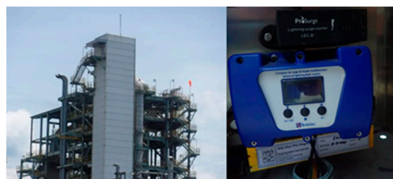
Figure 11. Installation of measurement system in refinery structure.
