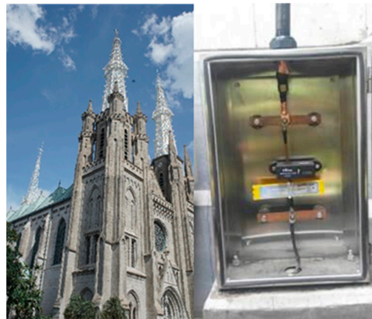
Figure 14. Installation of measurement system in a church.
