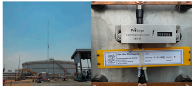
Figure 17. Installation of measurement system in tank area.
