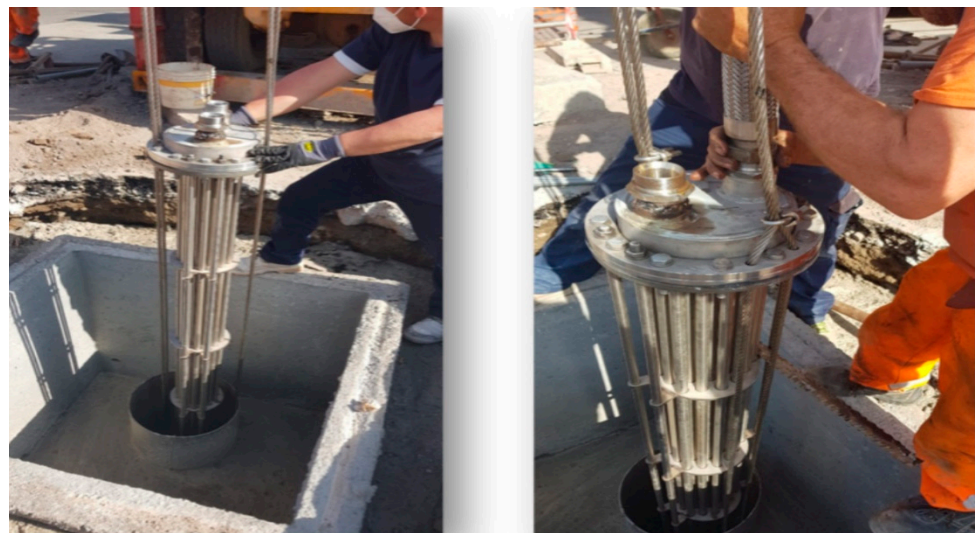
Figure 8. Installation of the DHE inside the geothermal well.
