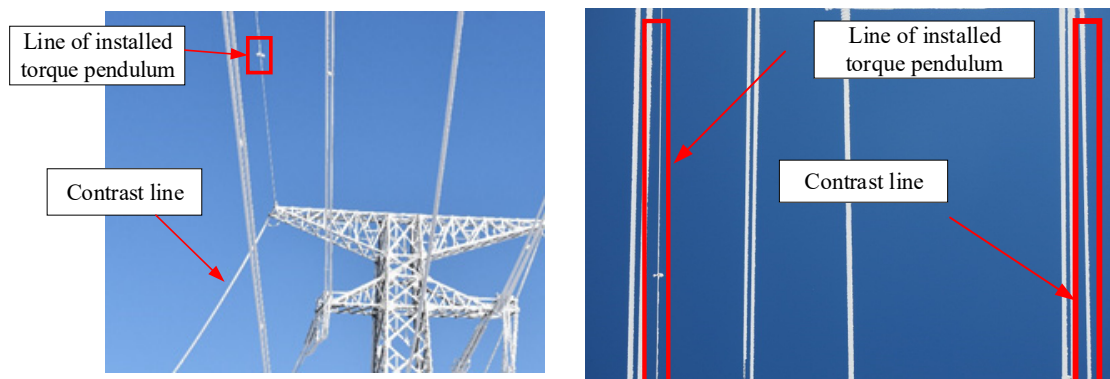
Figure 11. Natural icing contrast of overhead ground line.
