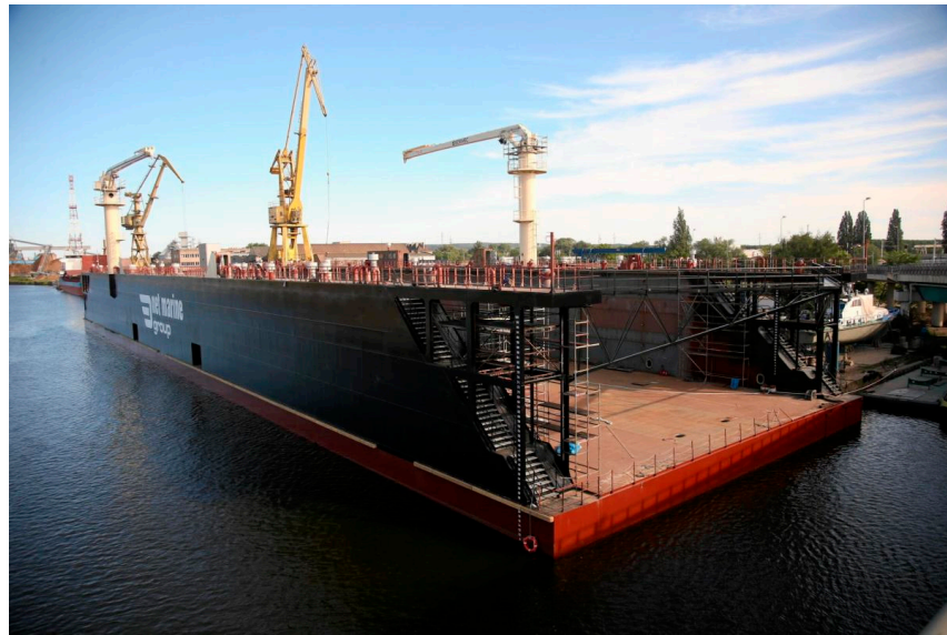
Figure 1. Floating dock at the Pomerania Ship Repair Yard [1].
