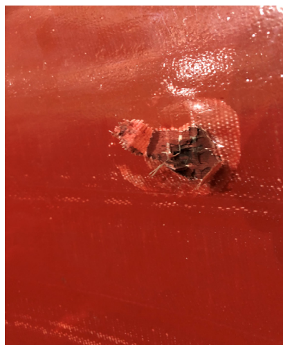
Figure 26. Winding breakdown after voltage test of transformer with unoptimised winding structure.
