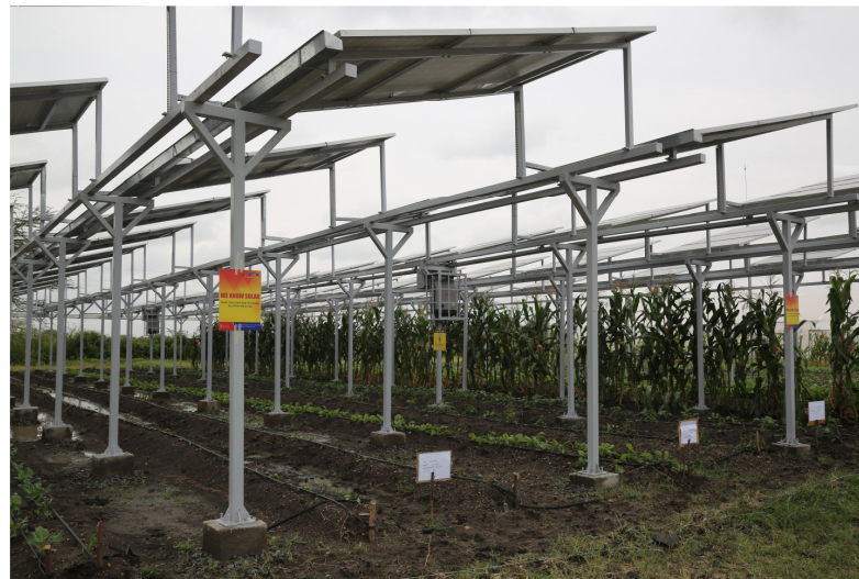
Figure 2. An image of a ground-mounted, fixed, overhead agrivoltaic system. The system is structured so that PV modules are, in general, separated enough from each other and sufficiently far from the ground to minimize shadowing effects. Photo courtesy granted under creative commons license by: Stacey Kihui/ICRAF [5].
