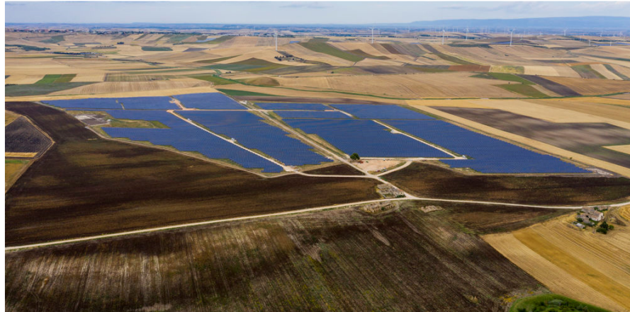
Figure 1. The largest Italian fixed-tilt ground-mounted utility photovoltaic plant. The 103 MW solar park is in Troia, Puglia, in an area previously dedicated to cropland activities. It was completed in 2021 and installed over an area of about 150 hectares with a power density of about 70 \text{ W/m}^2 . Photo courtesy granted by PV Magazine [2].
