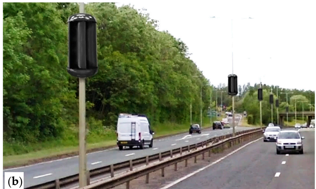
Figure 21. (a) Operation scheme of the Alpha 311 turbine, (b) application of Alpha 311 turbines in the road's median, properly designed to be retrofitted to existing infrastructure such as streetlights alongside roads. (Reprinted with permission from Ref. [129]. Alpha 311 Ltd., Kent, UK) [129].
