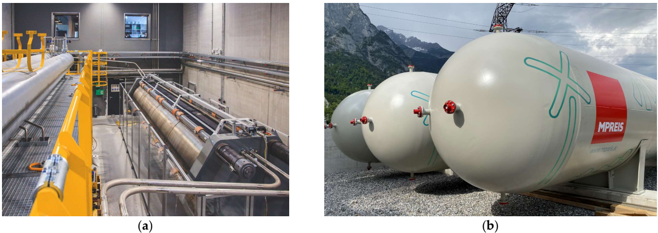
Figure 7. (a) PAE supplied by Sunfire GmbH at the right and the gas separators at the left; (b) three hydrogen storage vessels supplied by APL GmbH (Tyrolean company), with permission from MPREIS.
