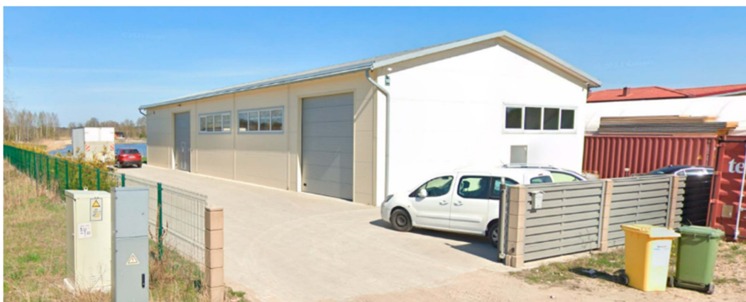
Figure 1. The industrial building used as a test facility.
