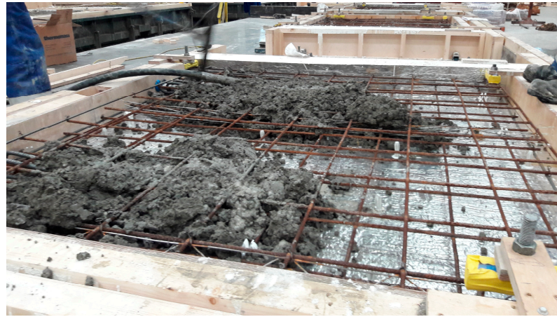
Figure 6. PCM–concrete composite panel under construction.
