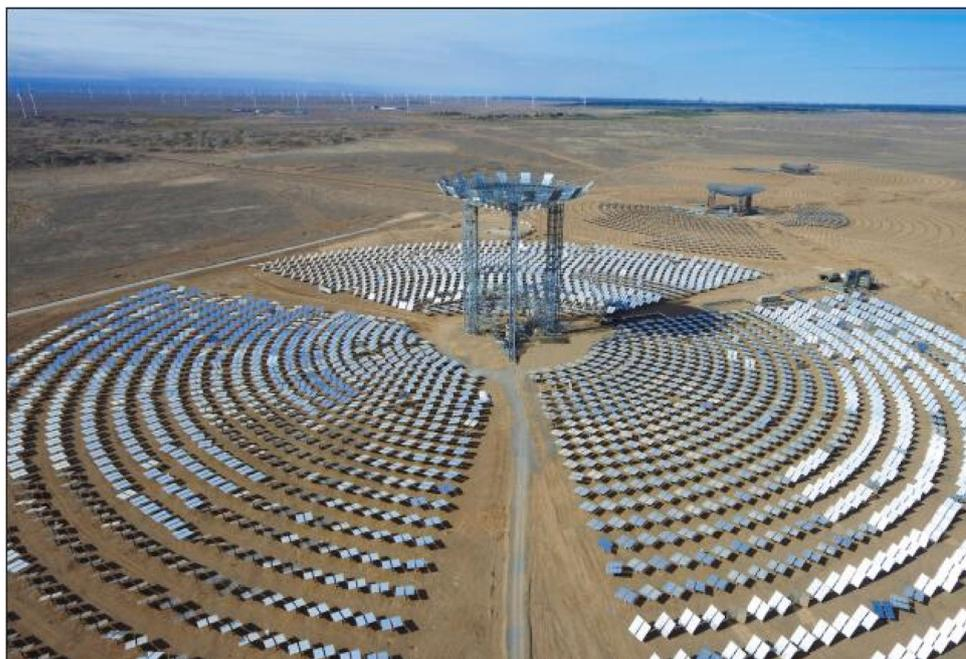
**Figure 33.** The beam-down CSP in Yumen Xinneng/Xinchen. Reproduced by kind permission of Elsevier from [196].
