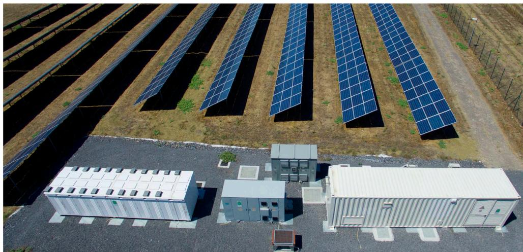
**Figure 25.** Example of battery energy storage system (BESS).
