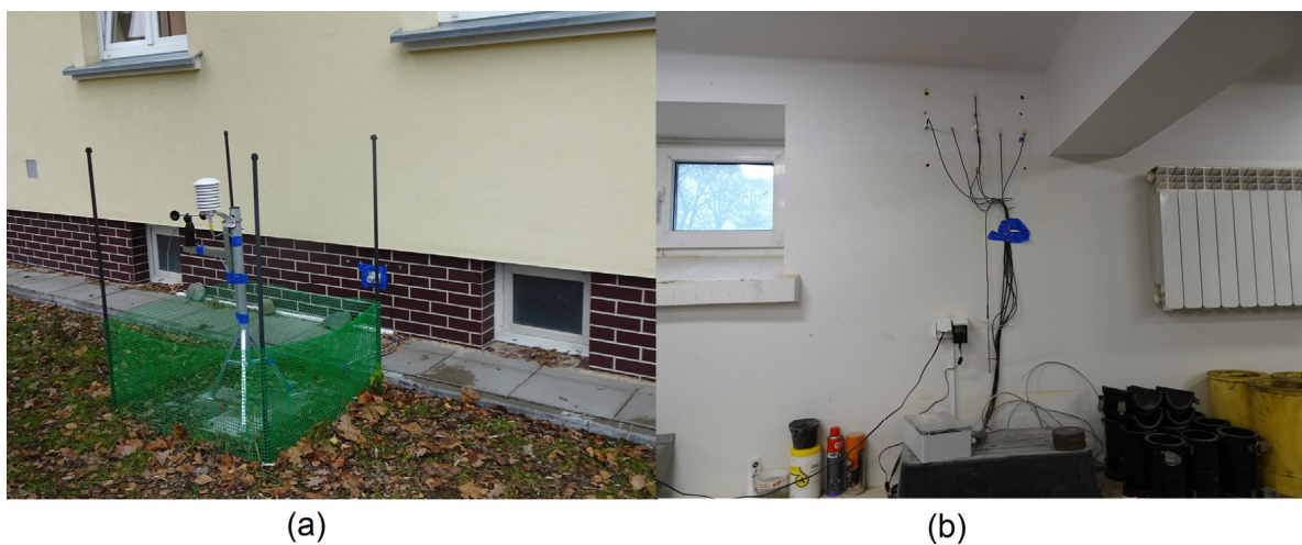
Figure 2. Photos of the measurement station: (a) external conditions sensors, (b) sensor holes in the wall.
