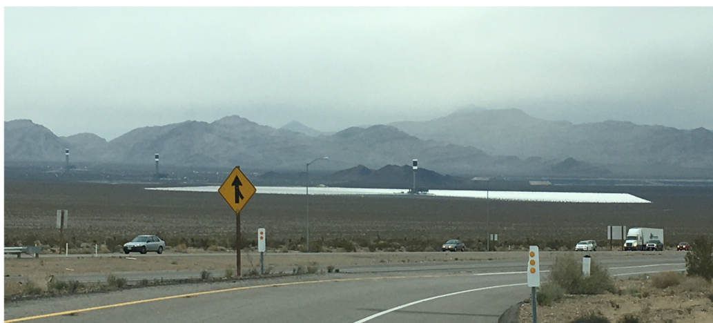
Figure 5. Ivanpah Utility-Scale Central Receiver Facility. Photograph by primary author.
