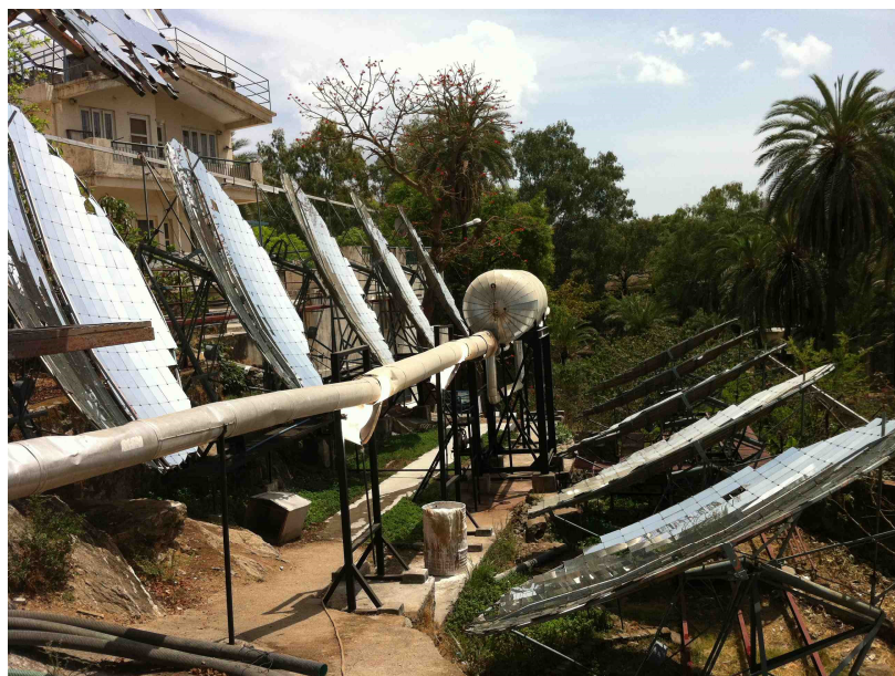
Figure 3. A Scheffler dish system at Brahma Kumari Headquarters, Rajasthan, India. Dual-sided receivers are under the steam tube. Photograph by the primary author.
