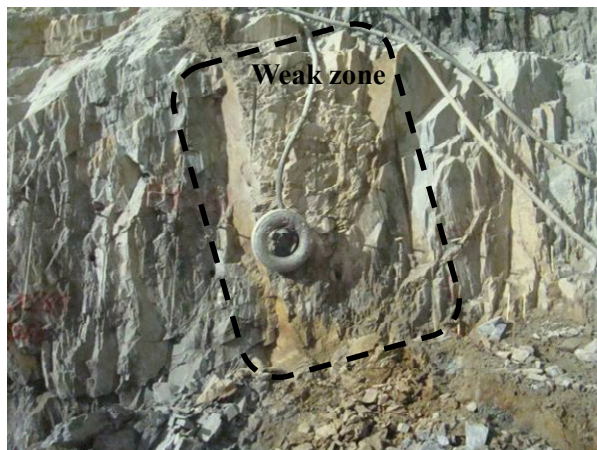
Figure 15. Weak zone of the section R0+263 at the main powerhouse.
