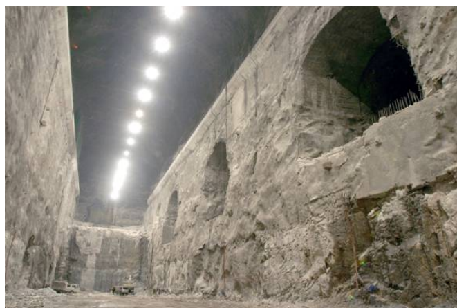
Figure 7. Photo of the excavated underground powerhouse of the Laxiwa hydropower station.
