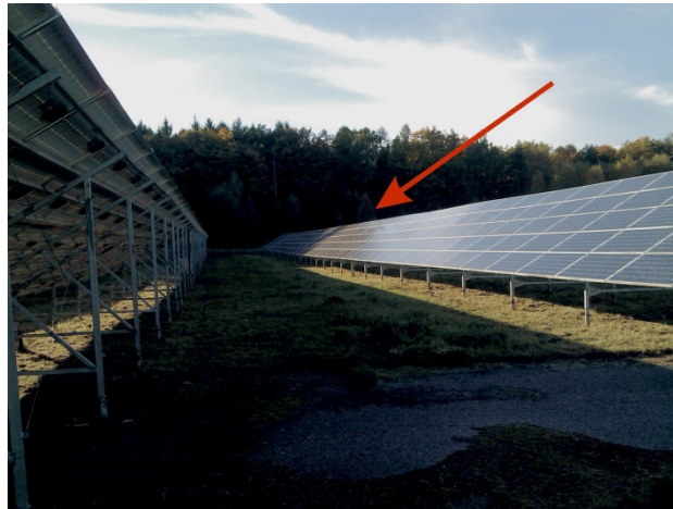
Figure 12. Trees overshadowing the section of the PV plant [25].
