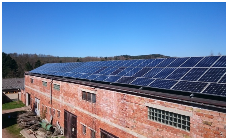
Figure 15. Selected part of the 100 kWp PV plant [27].
