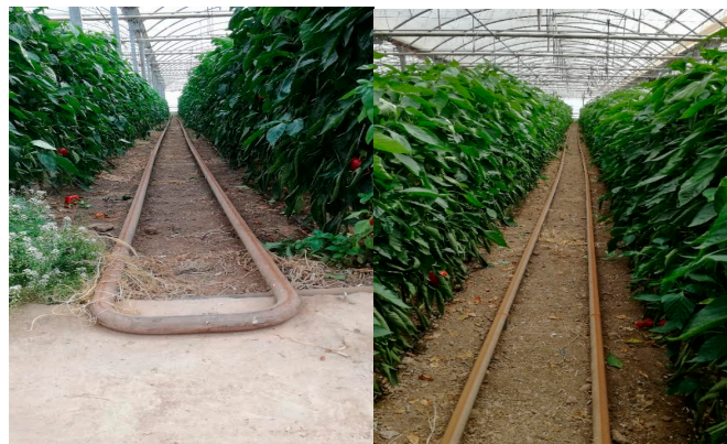
Figure 7. Steel plumbing system for distributing water vapor.
