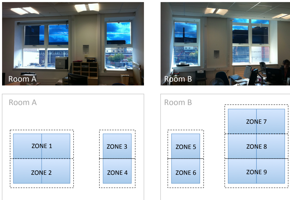
Figure 1. Photographs of the electrochromic (EC) windows in the two offices with corresponding schematics showing the control zones.
