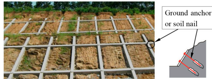
Figure 1. A typical application of grid beam structure on man-made slope.
