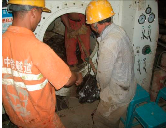
Figure 1. Soil sampling at the tunnel face.
