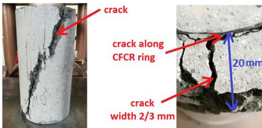
Figure 6. Typical failure mode of the HPSCFRC (high-performance self-compacting fibre-reinforced concrete) with a CFRP ring.
