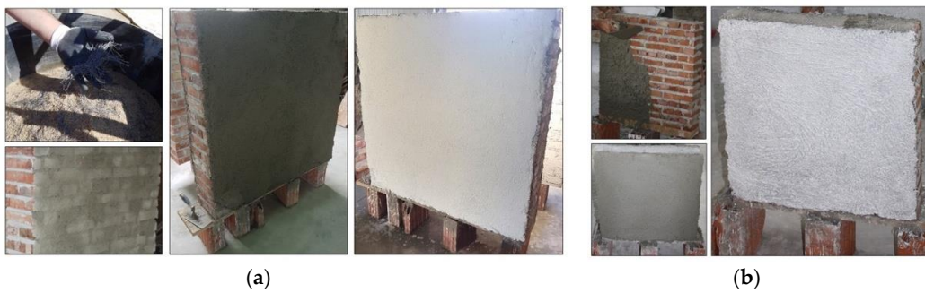
Figure 12. Application of the retrofitting with polypropylene fibers: (a) full-scale (W-series) and (b) half-scale panel (SW-series).
