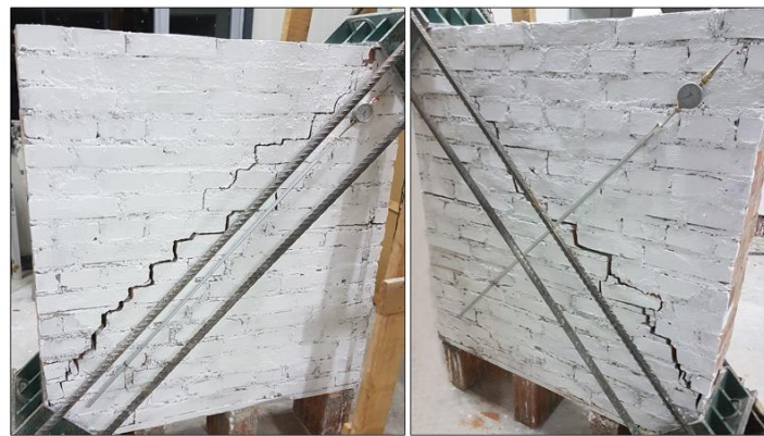
Figure 13. Failure mode of wall panel W-1-URM.
