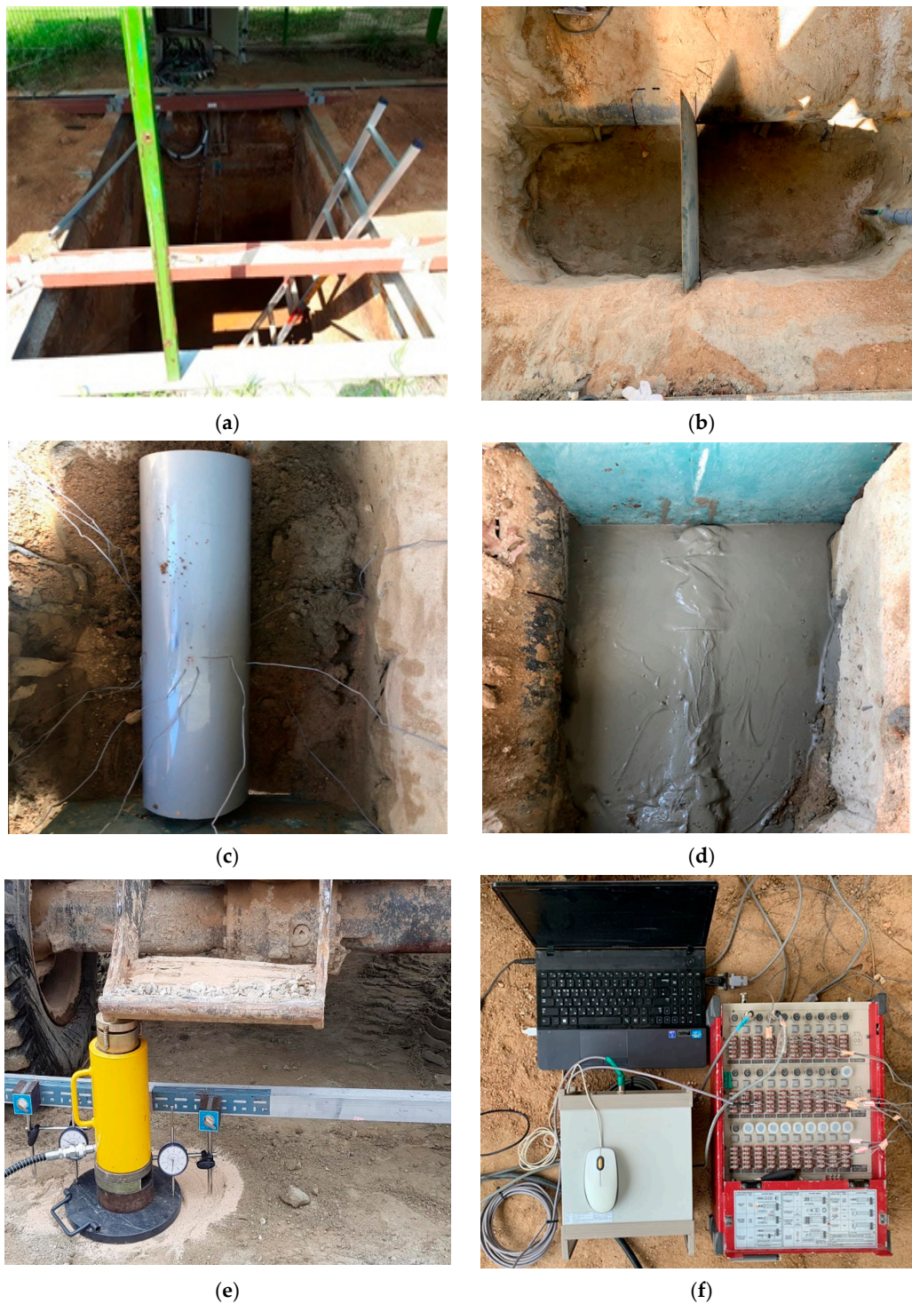
Figure 12. Plate bearing test procedure: (a) ground excavation and soil box installation; (b) ground construction; (c) buried sewage pipe; (d) CLSM construction; (e) plate bearing test; (f) test measurement.
