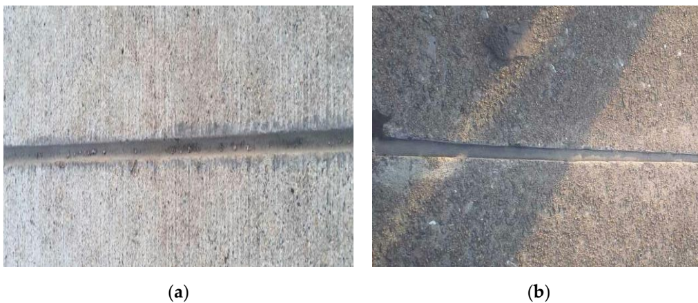
Figure 16. The appearance of the PCFC after two years. (a) The military airport in Tibet. (b) The military airport in Guangdong province.
