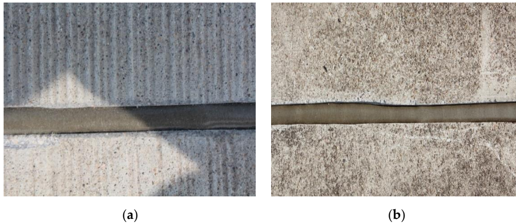
Figure 15. The appearance of the PCFC after 28 days of curing. (a) The military airport in Tibet. (b) The military airport in Guangdong province.
