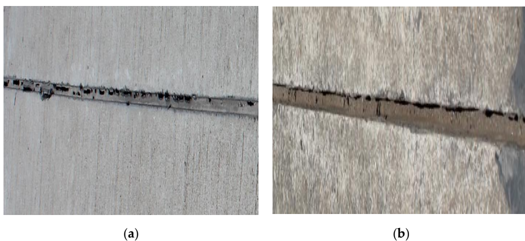
Figure 17. The appearance of the conventional joint sealants after one year. (a) The military airport in Tibet. (b) The military airport in Guangdong province.
