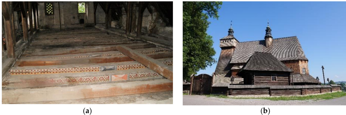
Figure 1. (a) The beam ceiling of the Gorzanów Palace—high humidity of the elements resulted from long-term leakage in the roofing; (b) The church in Haczów—repeatedly flooded by floods.
