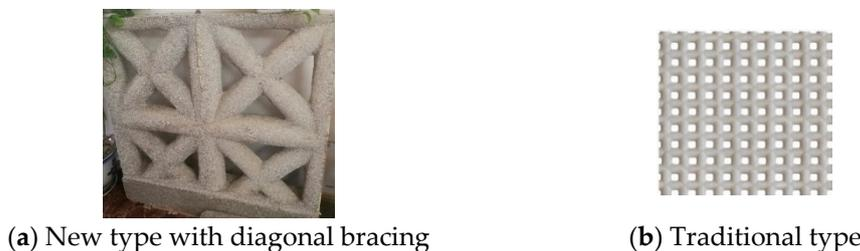
Figure 2. The skeleton of the latticed concrete wall.
