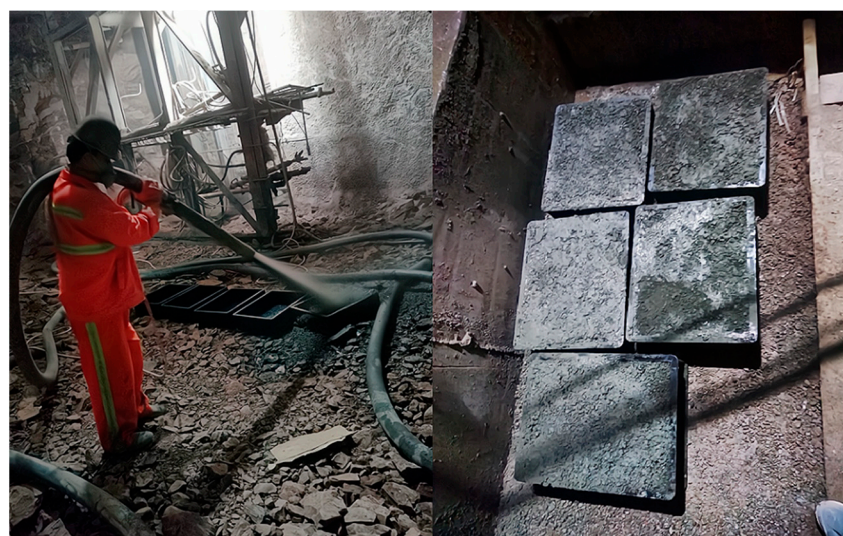
Figure 3. The preparation of on-site shotcrete slab.
