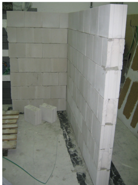
Figure 1. View of the wall before plastering.
