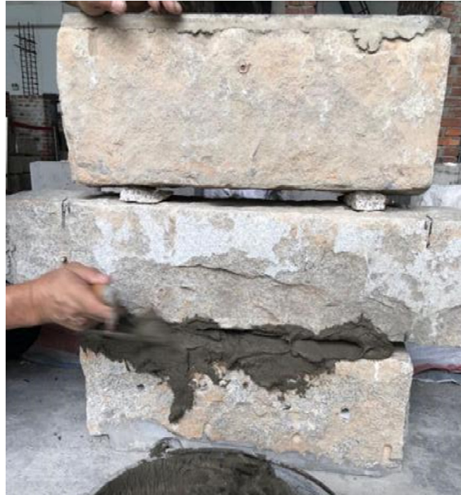
Figure 4. Filling the joints with mortar.
