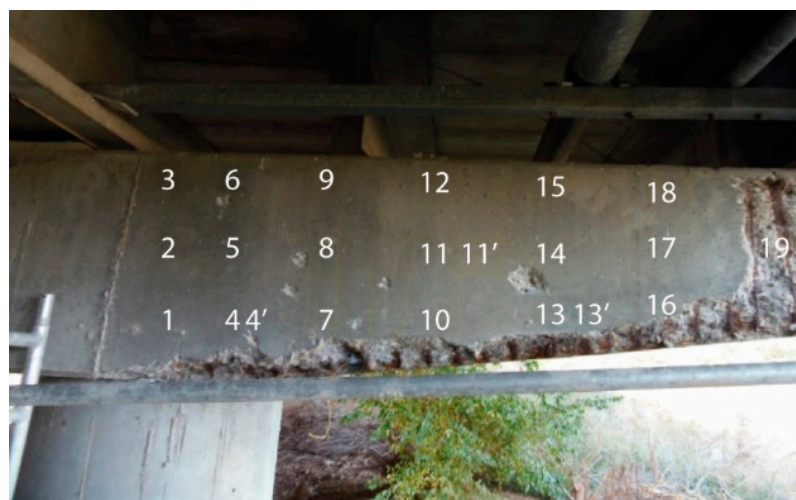
Figure 4. Points measured on the surface of the girder analysed (photo taken by S. Chinchón-Payá).
