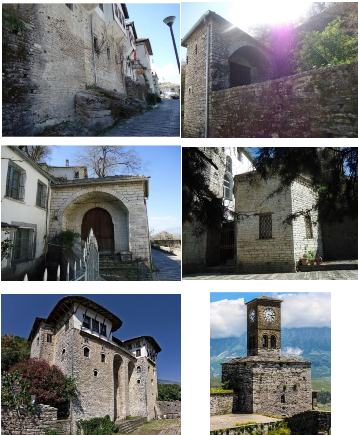
Figure 13. Several typical stone masonry buildings of Gjirokaštër.
