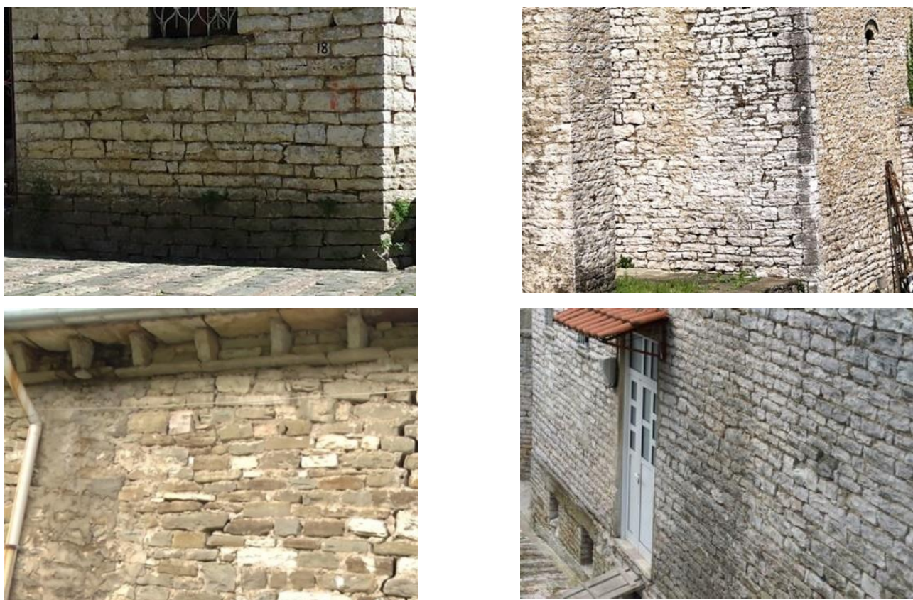
Figure 15. Typical stone walls of Gjirokastrë.
