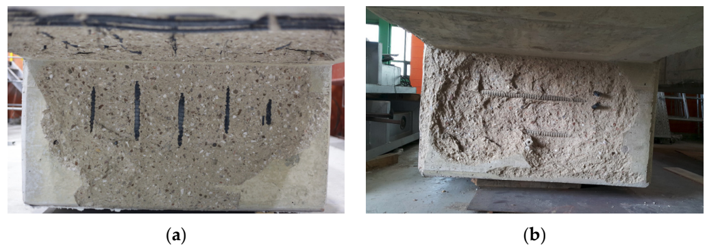
Figure 9. The exposed surface of wall-slab specimen after the fire test (3 h): (a) One-side heating (OS); (b) two-side heating (TS).
