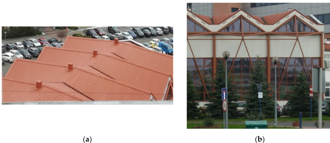
Figure 5. The external views of two opposite elevations of the experimental hall at a university roofed with the shell structure: (a) the roof structure; (b) the south side of the entire building.
